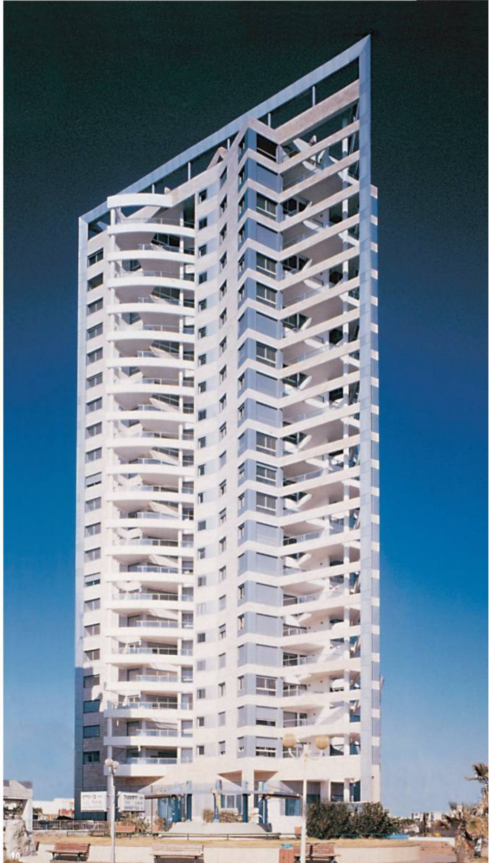
Arena Residence, Stage One - Bat Yam
